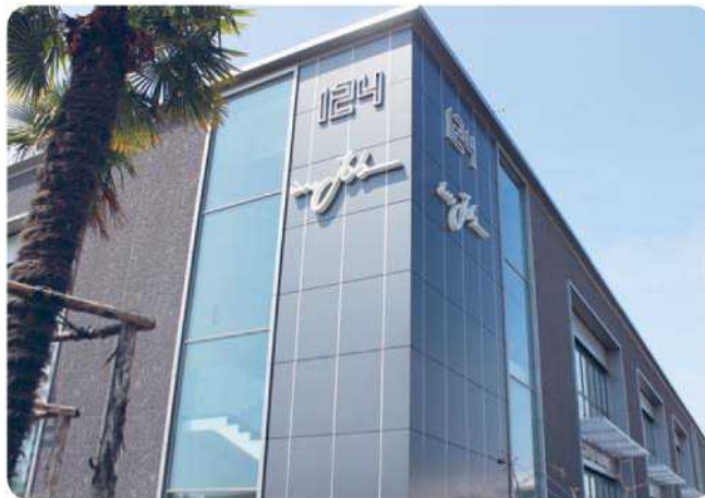
Headquarters in job
